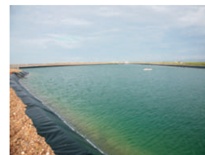
Water reservoir (photo A. Enamorado)
